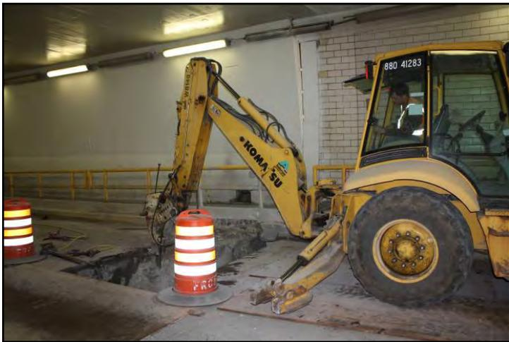
*Contractor removed concrete to expose joints below roadway surface for grouting and sealing.*
