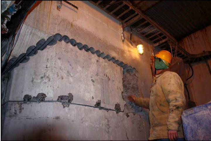
*Photo shows holes cored and wire-saw cuts made by the contractor in one of the recesses prior to removing the concrete in large blocks.*
