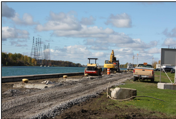
Paving and mooring button rehabilitation at the upper guidewall at Snell Lock
