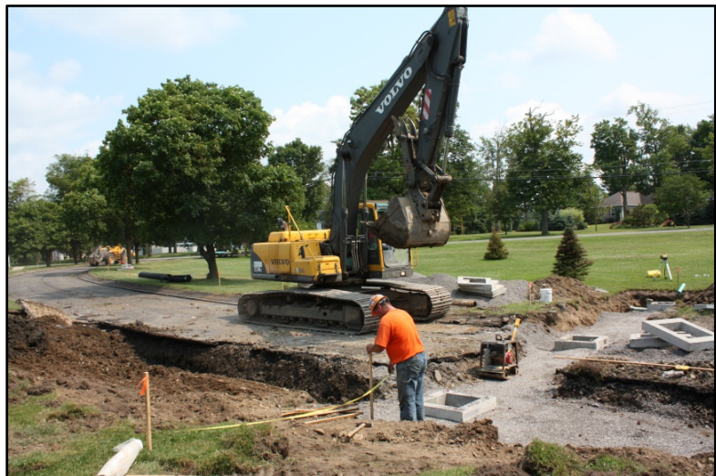
J.E. Sheehan Contracting replaces severely deteriorated sidewalks and roadways at the front entrance of the SLSDC's Administration Building in the Village of Massena.
