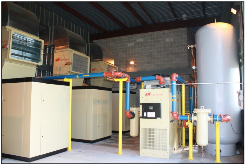
Newly-installed compressor system at Snell Lock. A similar system was also installed at Eisenhower Lock. The compressors are used for maintenance work, and for controlling ice in and around the locks, as needed.
