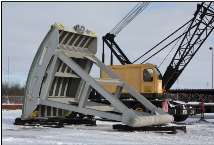
One of the new single-skin culvert valves just prior to its installation on the south side of Snell Lock following the 2010 navigation season.
