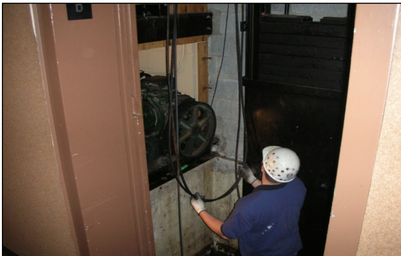
ThyssenKrupp Elevator Co. worker prepares cabling for elevator modernization in the SLSDC's Administration Building.
