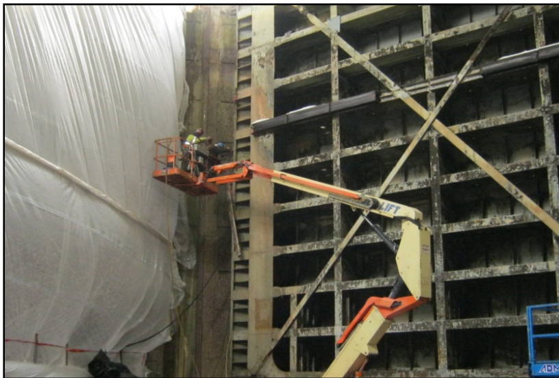
Workers assess the condition of the Eisenhower Lock upstream miter gate prior to removing the gate for rehabilitation work.
