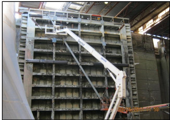
Hohl Industrial Services, Inc. installs new diagonals on the Eisenhower Lock upstream miter gate as part of the project.
