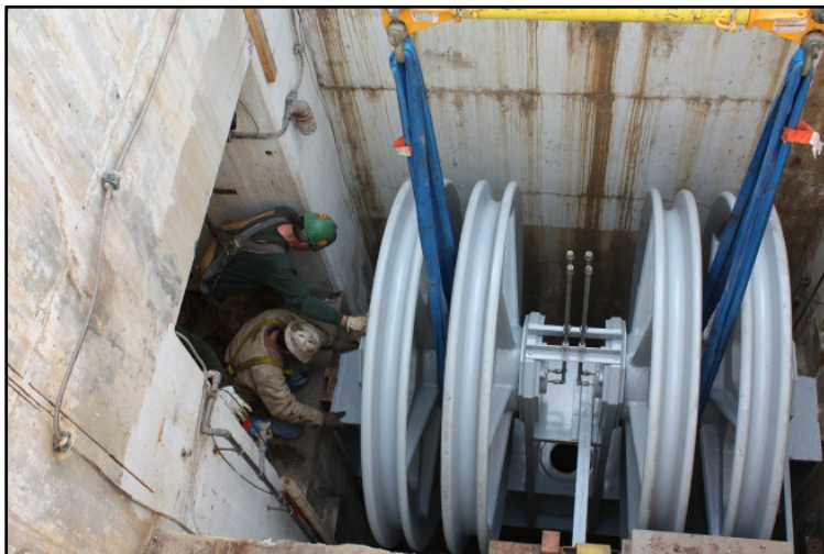
B.S. Industrial Contractors, Inc., workers reinstall the vertical lift gate rope wire sheaves at the Eisenhower Lock.
