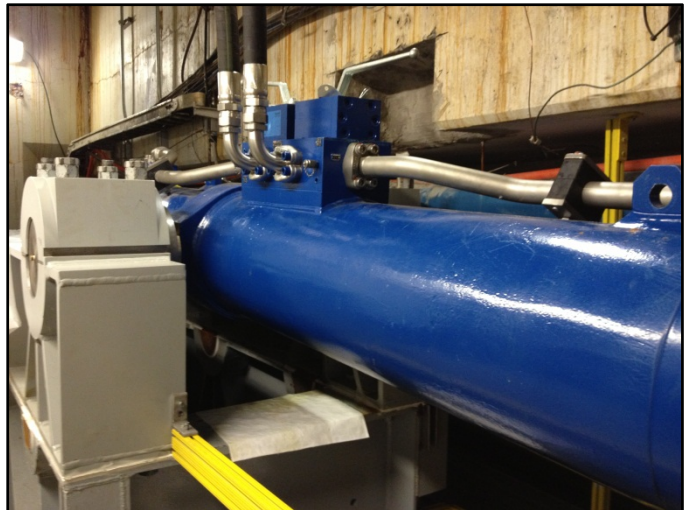
The SLSDC's new hydraulic-based culvert valve machinery unit. A total of eight units have been or will be installed at the two U.S. Seaway locks.
