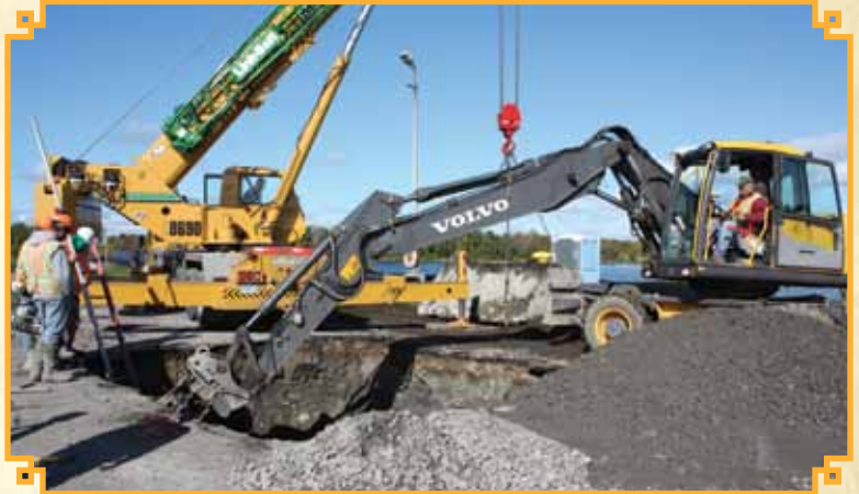
Resetting the mooring buttons on the upper guidewall of Eisenhower Lock before repaving.
