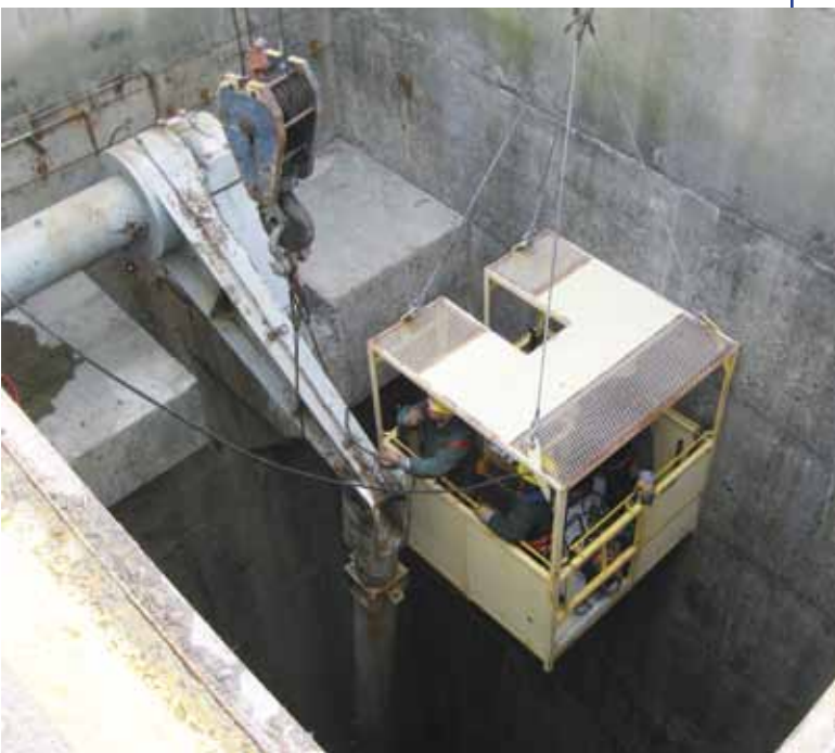
SLSDC maintenance personnel disconnecting strut in preparation for replacing the upstream south filling valve and strut at Snell Lock with a new single valve and strut.
