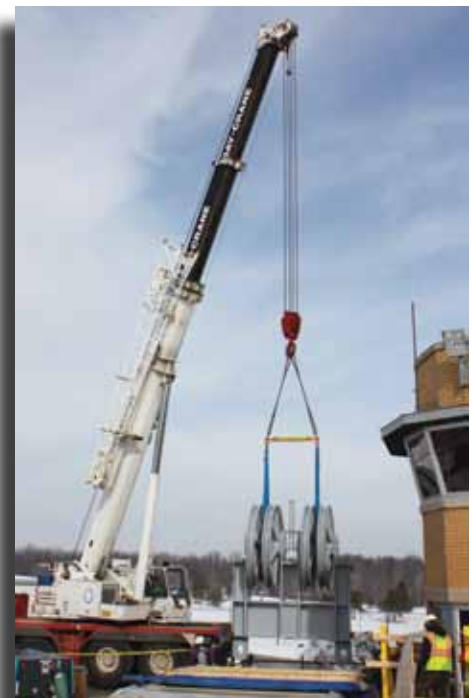
Contractor re-installing refurbished sheaves and support frame for the emergency vertical lift gate at Eisenhower Lock.
