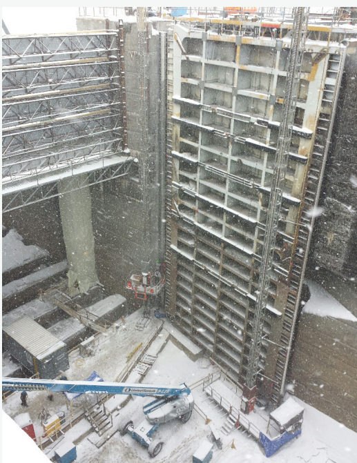
Miter gate rehabilitation work continued around the clock at the Snell Lock in Massena, N.Y.
