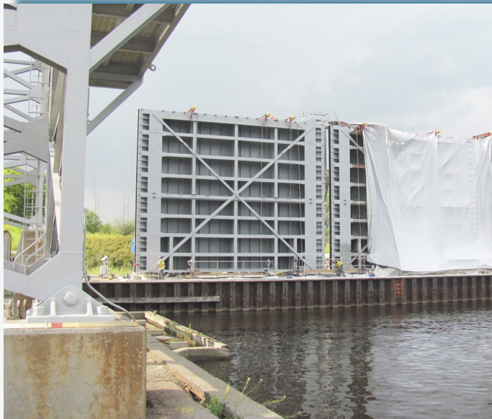
SLSDC contractor prepares to put the finishing touches on one of the cleaned and painted spare gate sections being stored at the SLSDC Snug Harbor.
