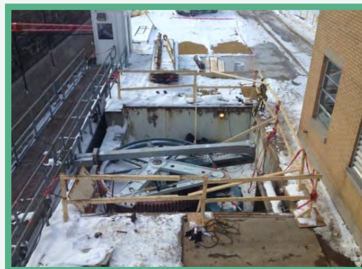
Rehabilitating the downstream miter gate gear drives at Eisenhower Lock in Massena, N.Y.
