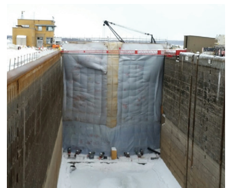
Blast cleaning and painting miter gates at Snell Lock. The contractor had to erect scaffolding and tarps to create a containment enclosure used to help control temperature and humidity conditions during the project.
