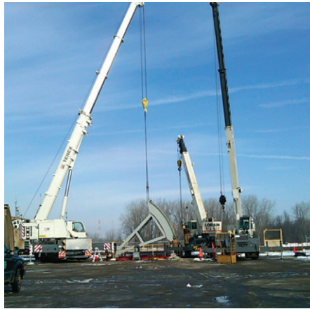
Modifying lock culvert valves at Snell Lock. SLSDC maintenance personnel were prepared for the critical lifts required to replace a filling/emptying culvert valve.
