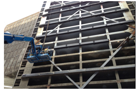
Eisenhower Lock miter gate rehab.
