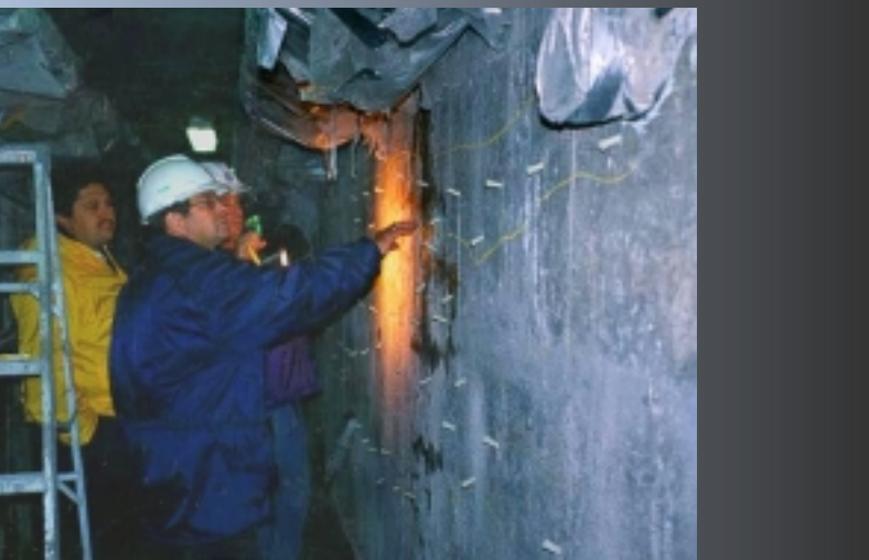
Crack Injection in the cable galleries, St-Lambert Lock
