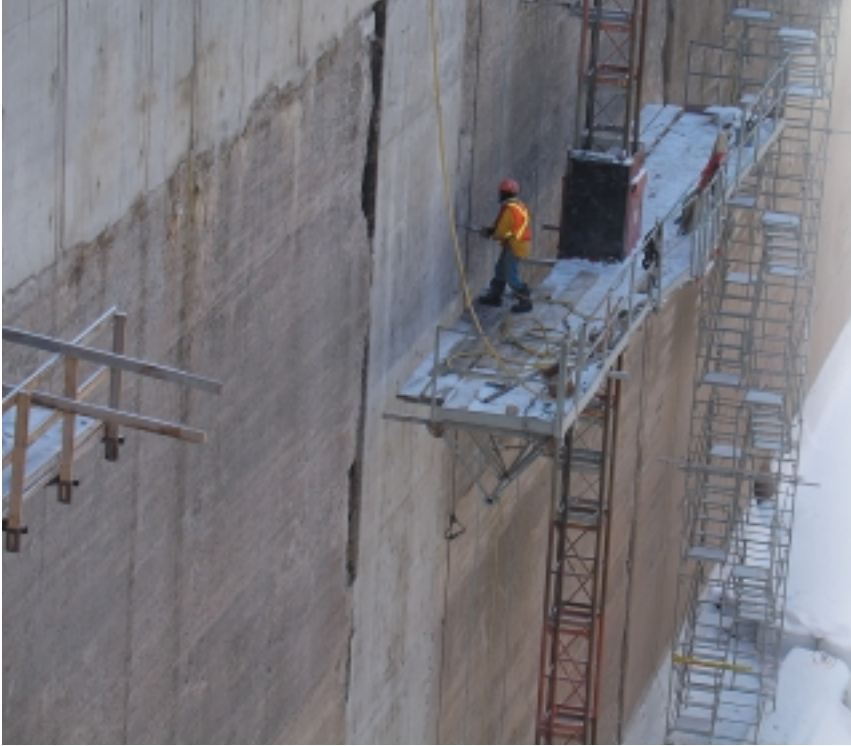
Contractor refacing lock wall during 2005 winter works
