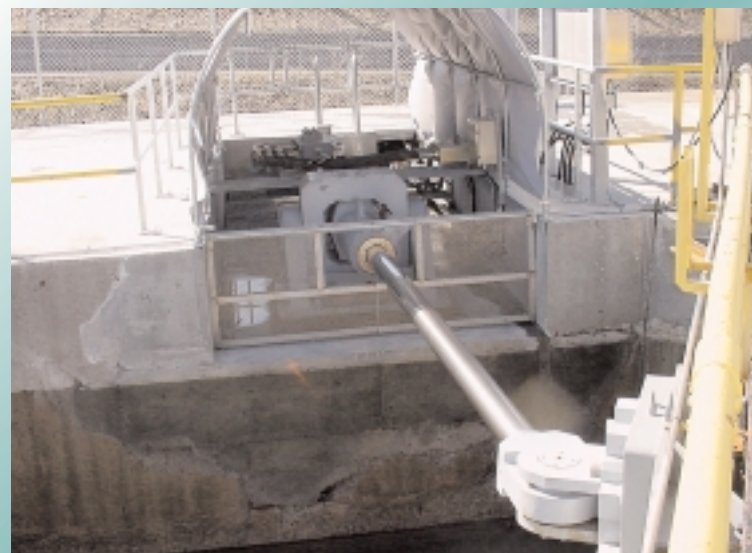
New Hydraulic Cylinder at Lock 7, Gate 4 Iqbal S. Biln
