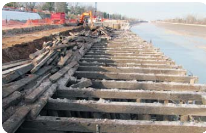
Before: Removal of timber tie up wall at Lock 2 (Welland Canal)
