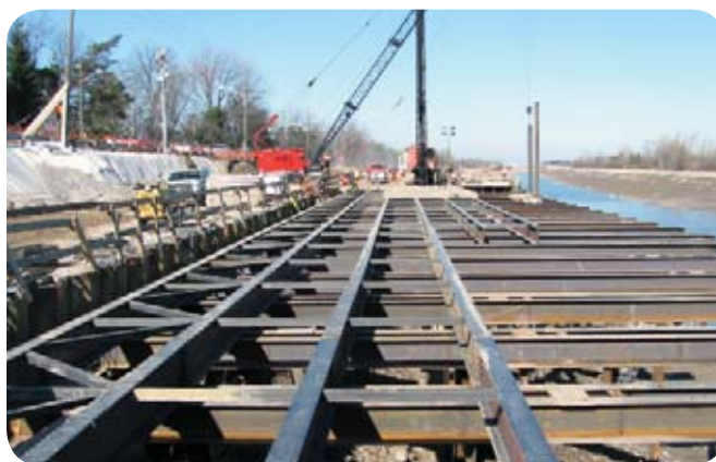
After: Construction of new tie up wall at Lock 2 (Welland Canal)
