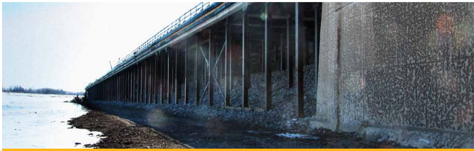
Completed section of a new tie-up wall within the Welland Canal
