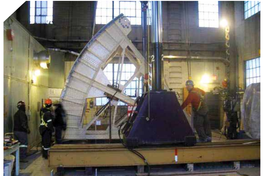
View of lock valve being re-installed after rehabilitation.
