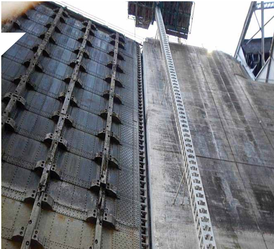
View of typical gate quoin repairs in the Welland Canal.
