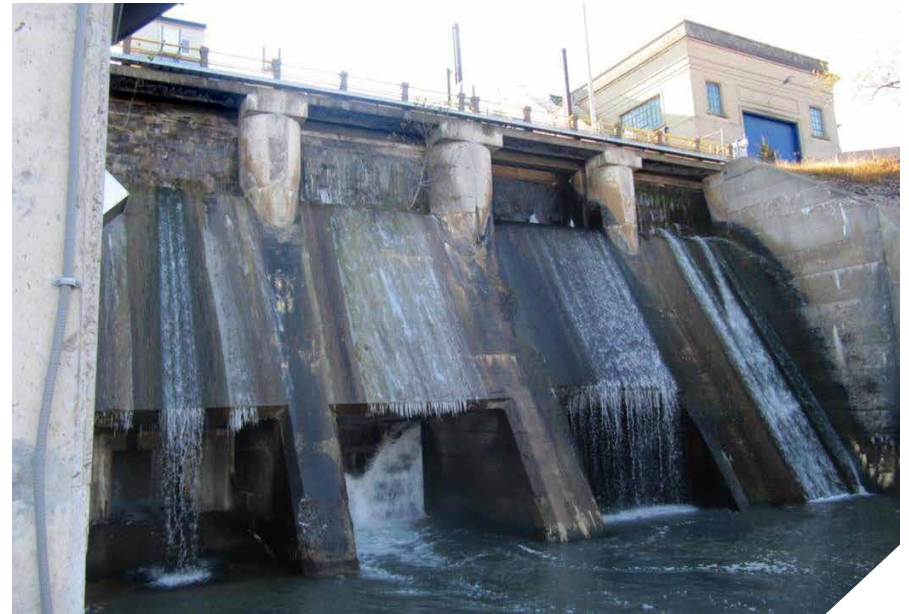
View showing weir valves in operation.
