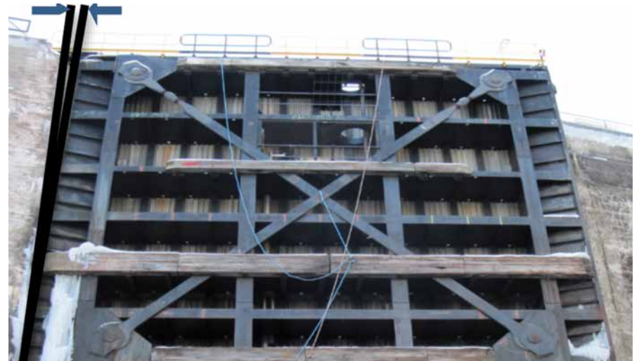
View of misalignment of the lower gates at Beauharnois Lock 3 prior to rehabilitation.
