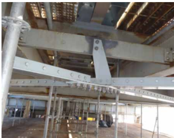
View of steel repairs underway at Bridge 3
