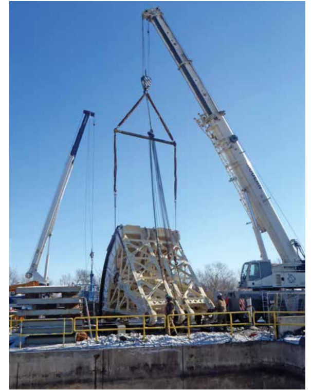
Installation of rehabilitated valve into the valve pit
