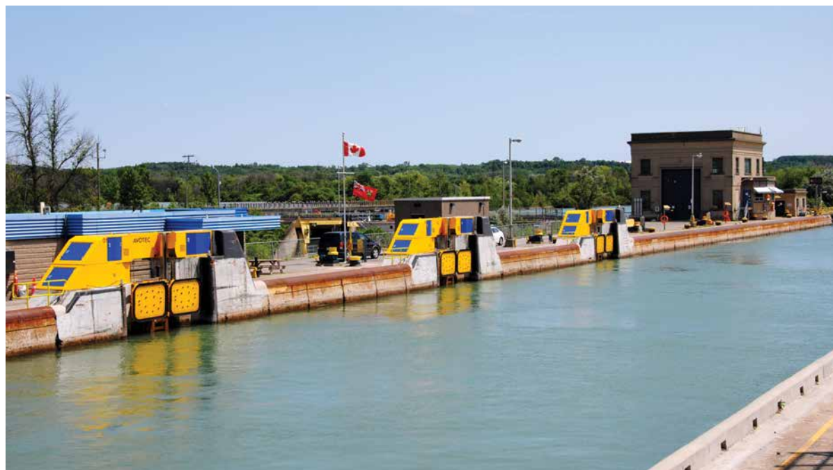
HFM pads standing ready to moor a ship at Lock 3 (Welland Canal)
