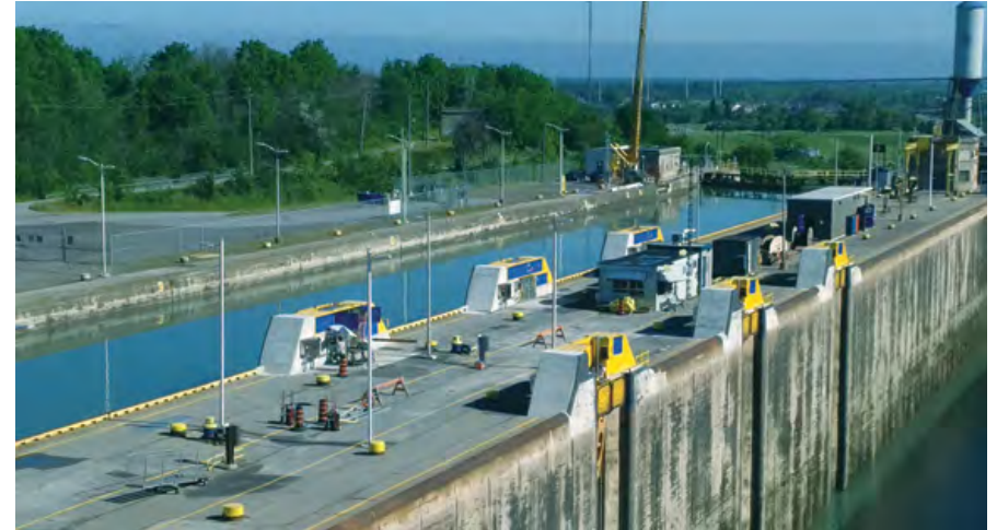
Hands-Free Mooring Equipment at the Flight Locks (Welland Canal)
