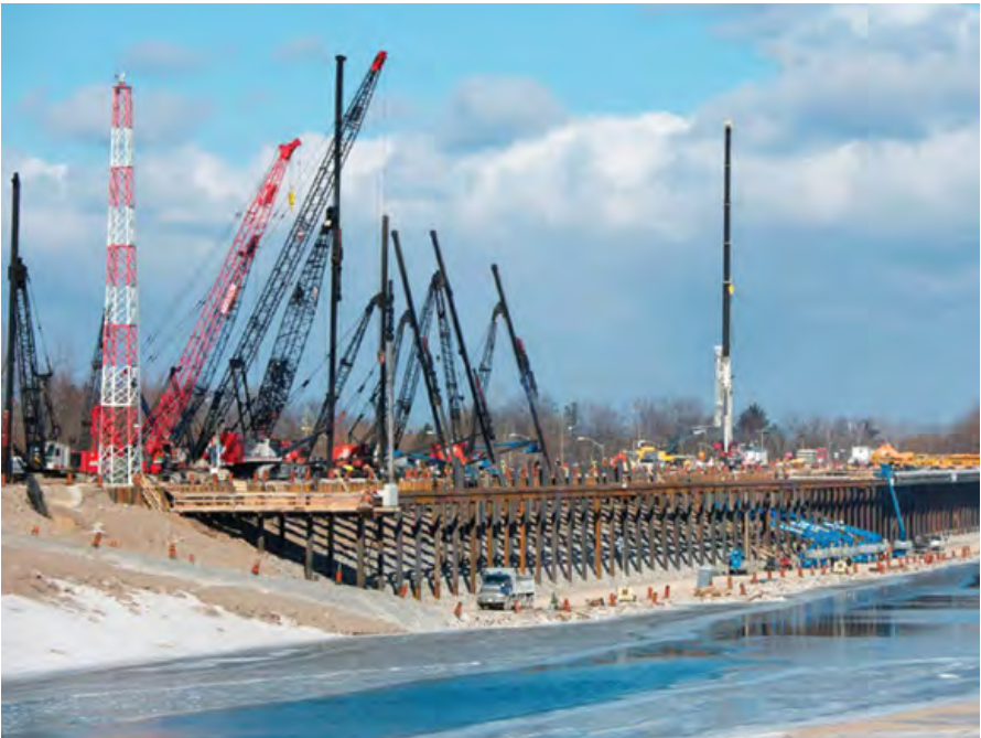
Photo of a portion of the 1.9 km of tie-up walls in the Welland Canal during the reconstruction process
