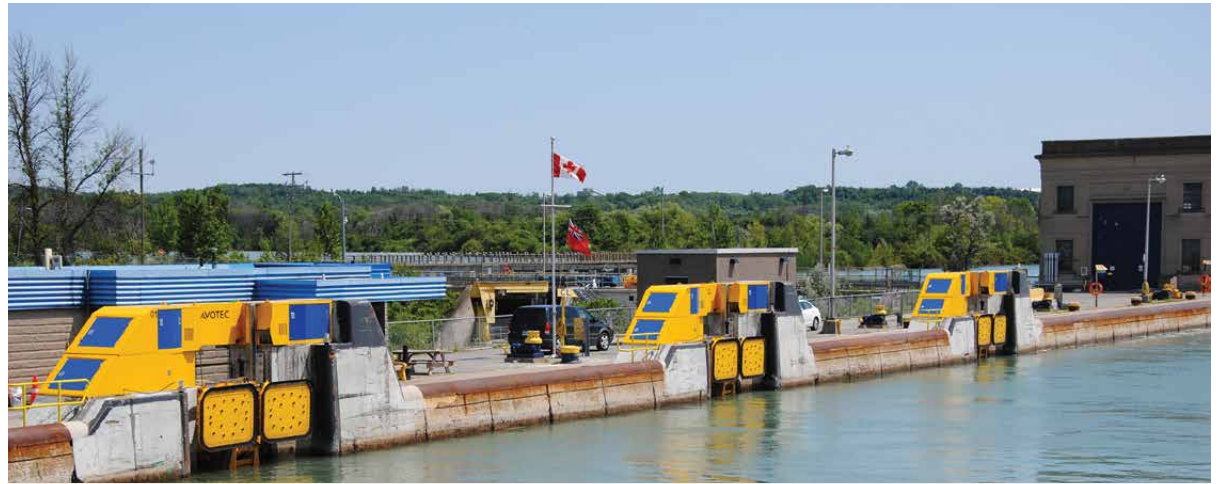
Each high-lift Seaway lock is equipped with three HFM units (Lock 8 in the Welland Canal and the Iroquois Lock, which serve as low-lift locks, are not equipped with HFM and utilize a "walk-thru" procedure for ships to go through the lock without tying up)
