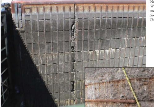
North Lock Wall at Snell with Vertical Wall Armor. (Note typical damage at monolith vertical joints) Source: Saint Lawrence Seaway Development Corporation
