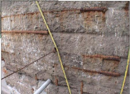
Concrete lock wall surface deterioration at Welland Canal Lock #7 (note exposed rebar at damaged area) Source: The St. Lawrence Seaway Management Corporation
