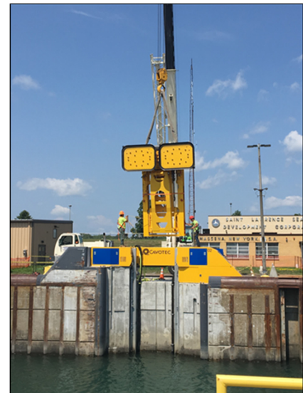
Work crews install the hands-free mooring units at Eisenhower Lock.
