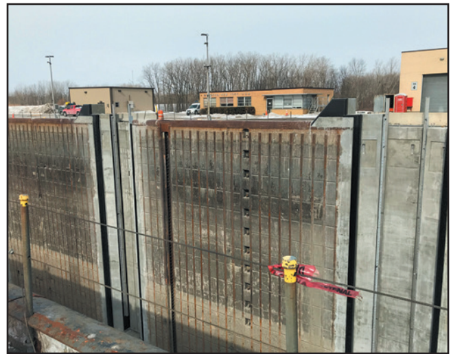
Completed HFM slots at Snell Lock.
