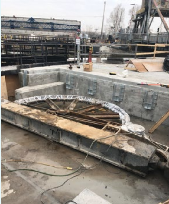
Côte-Ste-Catherine Lock 2 – Reconstruction of the protective covers for gear mechanisms at gates 5 and 6
