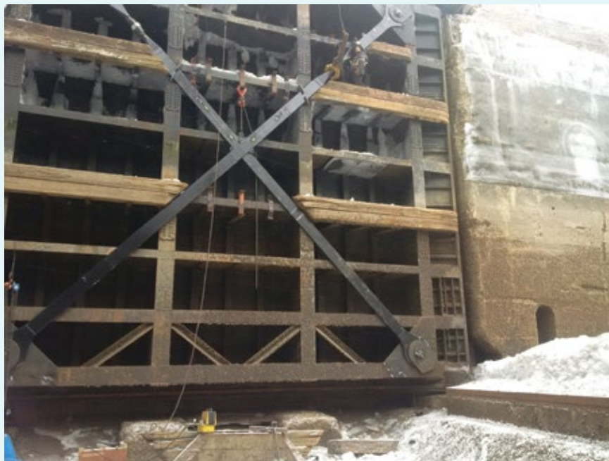
St. Lambert Lock 1 – Re-tensioning of diagonal braces on gates 7 and 8
