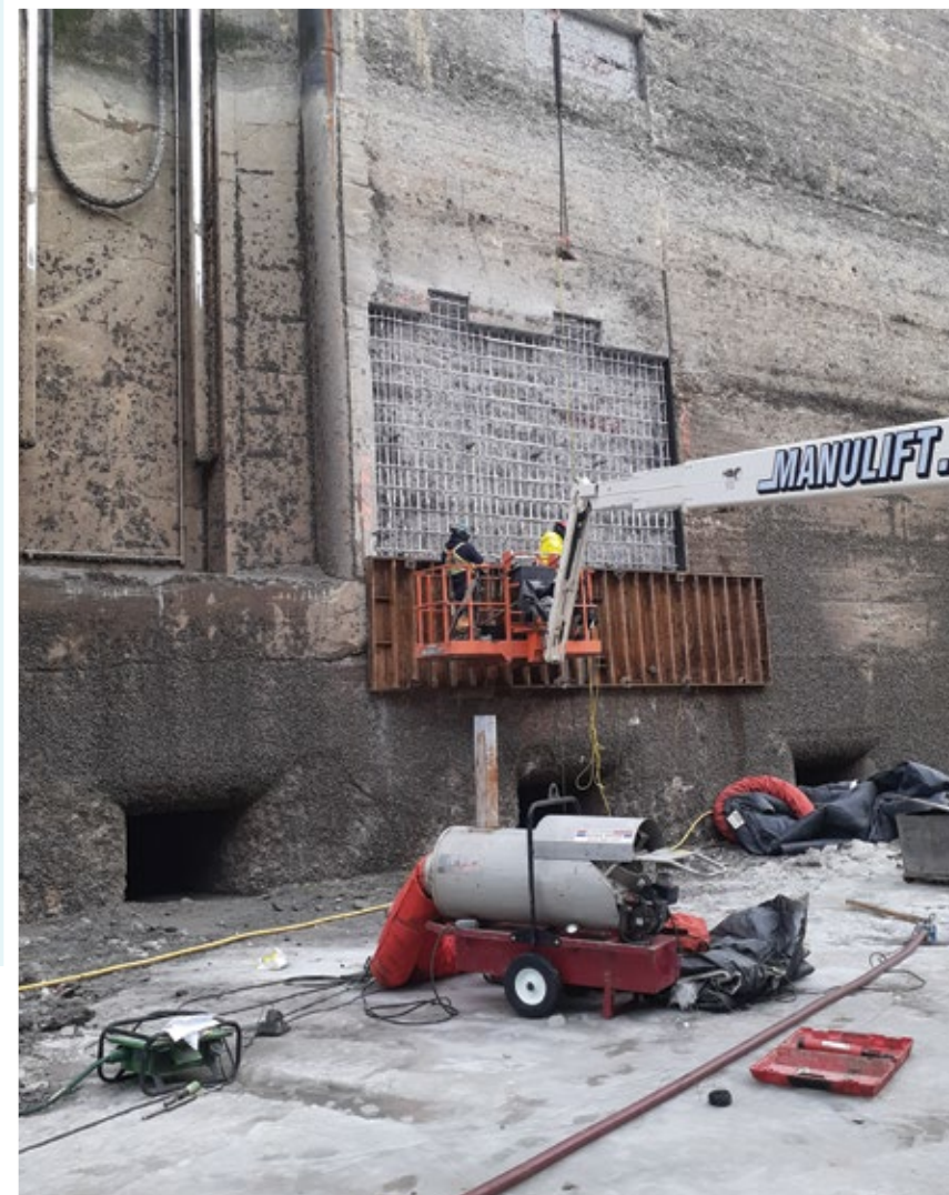
St. Lambert Lock 1 – Concrete repairs to the vertical wall surfaces
