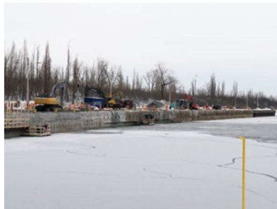
Côte-Ste-Catherine Lock 2 And Beauharnois Lock 3 – Reconstruction of the upper approach walls and installation of new fenders
