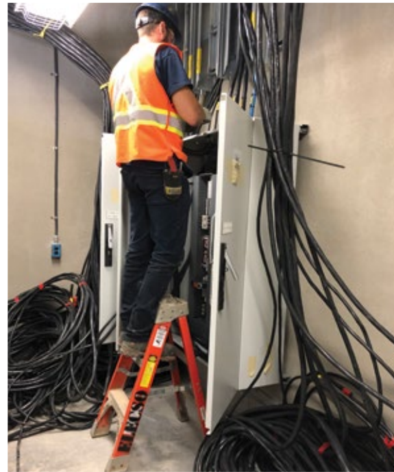
Beauharnois Lock 3 – Installation of new electrical panels and cables in four electrical rooms
