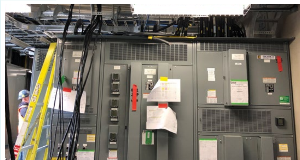
Beauharnois Lock 3 – Installation of new electrical panels and cables in four electrical rooms
