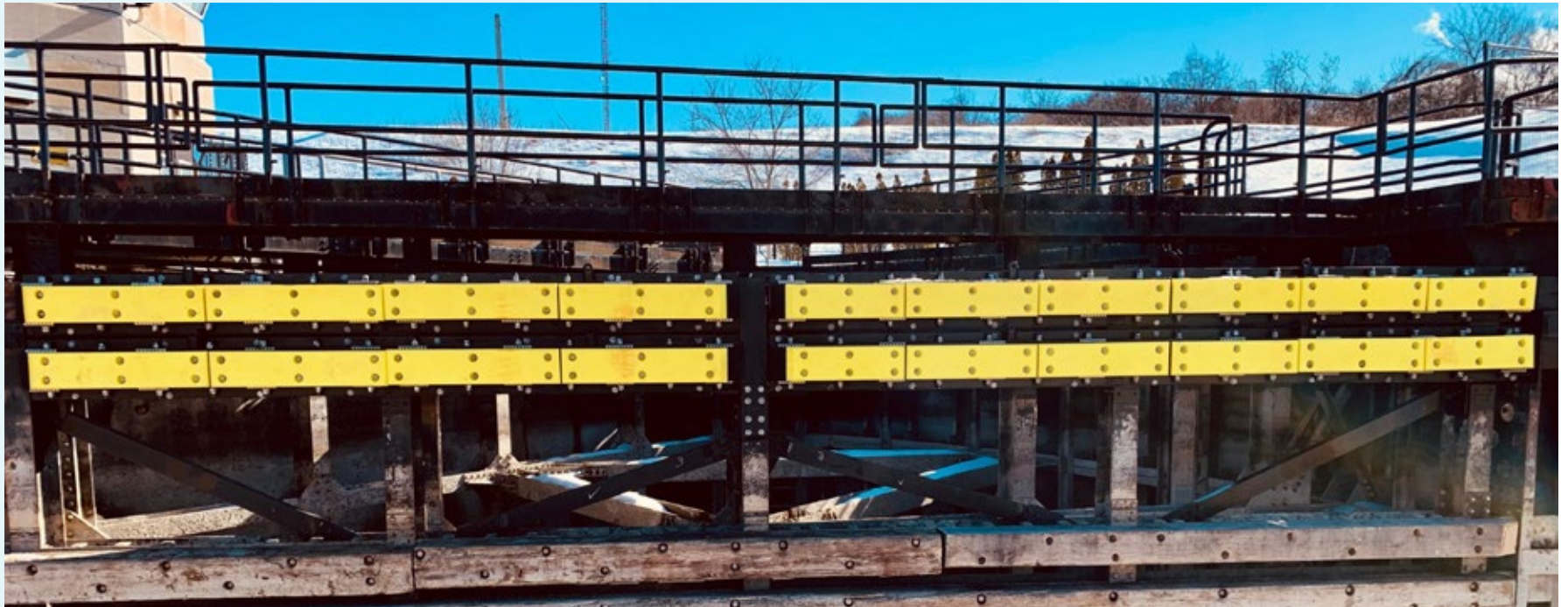
Iroquois Lock 7 – Replacement of the top wooden defense beams on lock sector gates, using a new type of material
