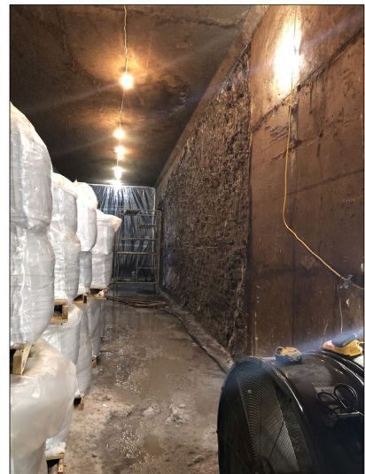
Recessed concrete walls prepared for rehabilitation during the winter months of FY 2019
