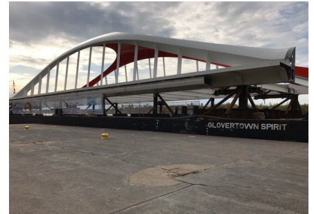
The Western half of the Commissioner Street Bridge transited through Snell Lock via the Glovertown Spirit barge.
