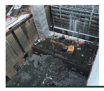
Above: Finishing demolition of Phase I diffusers at Eisenhower Lock.
