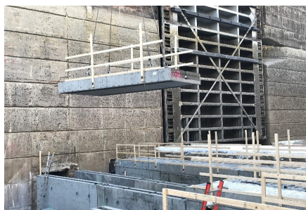
Lifting new precast concrete diffuser "cap" into place at Eisenhower Lock
