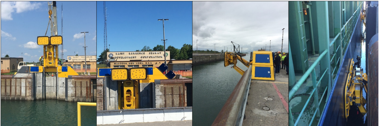
Hands Free Mooring unit fully operational at Eisenhower and Snell Locks
