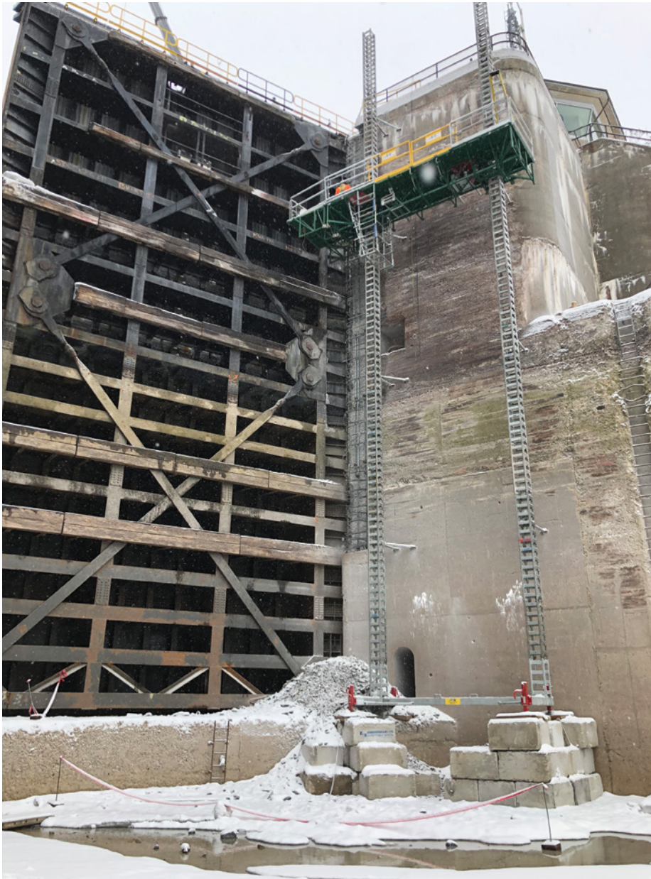
MLO - Lock 4, Wall Concrete Repairs and replacement of Miter quoins on G3&G4
