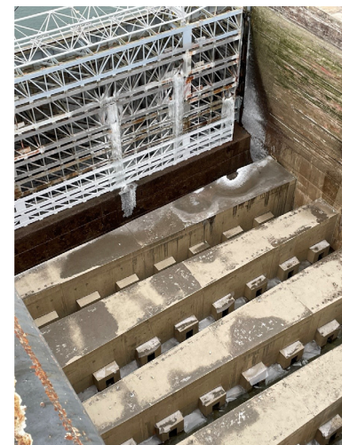
Eisenhower Lock Being Dewatered for 2023 Winter Work
