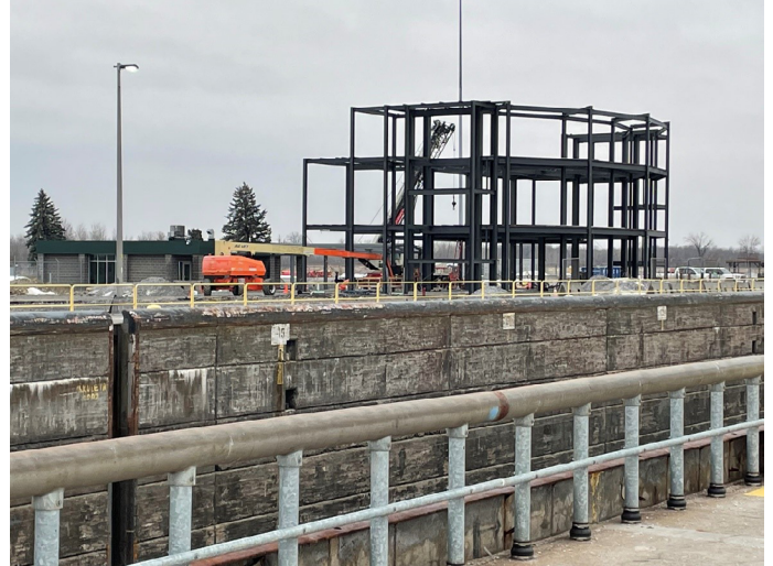
January 2023: New Visitor Center Structural Steel Being Erected
