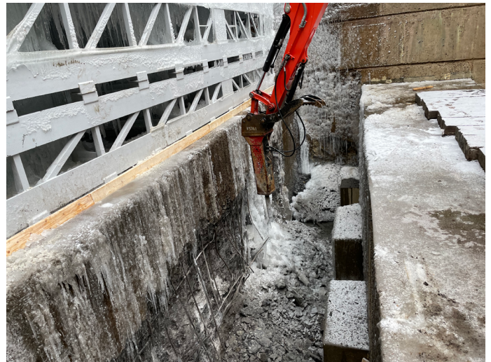
Eisenhower Concrete Demolition
