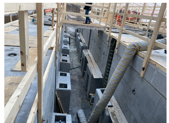
Snell Diffuser Structures Replaced
