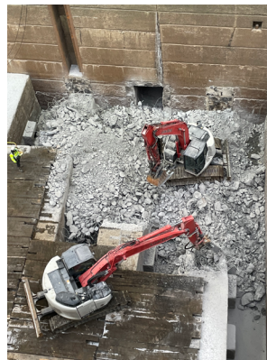
Snell Diffuser Structures During Demolition
