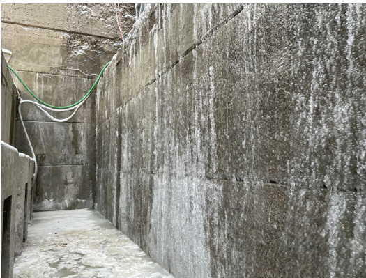
Eisenhower Concrete Repairs Made
