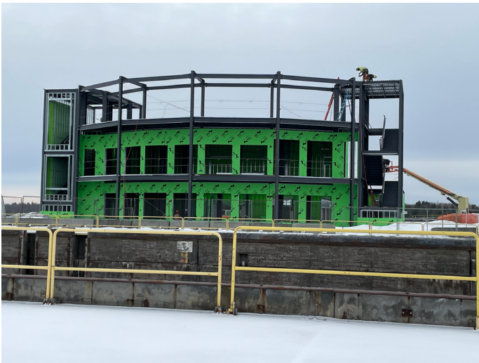
February 2023: New Seaway Visitor Center Construction Progress
