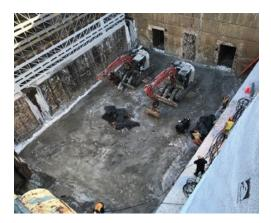
Finishing demolition of second phase diffusers at Eisenhower Lock.
