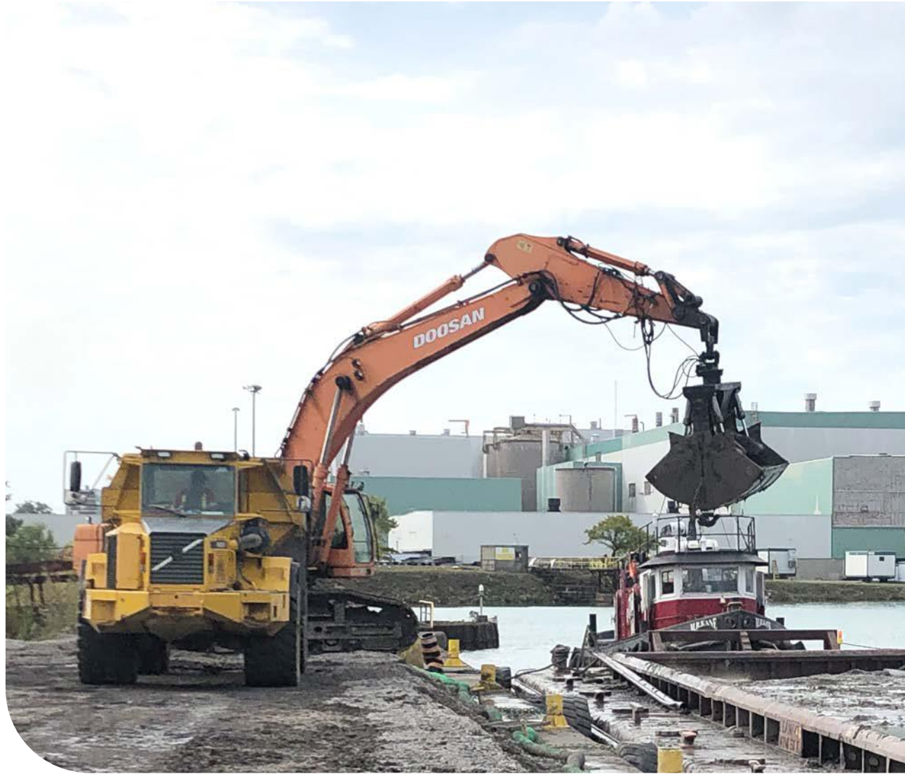
Off-loading Dredged Material at Tenant-Occupied Wharf
