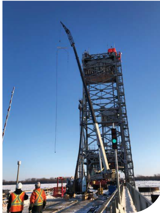
Replacement of counterweight cables on the St-Louis de Gonzague vertical lift bridge (near Salaberry-de-Valleyfield, Quebec)
