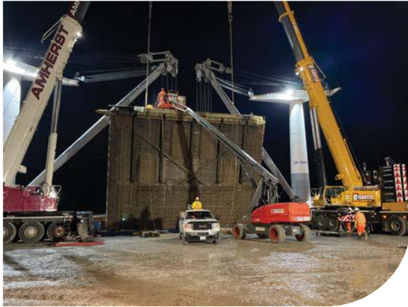
Welland Lock 8, complete removal of gates in anticipation of replacement
