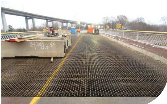
Replacement of the steel deck at the Queenston St. bascule bridge (Homer Bridge)
