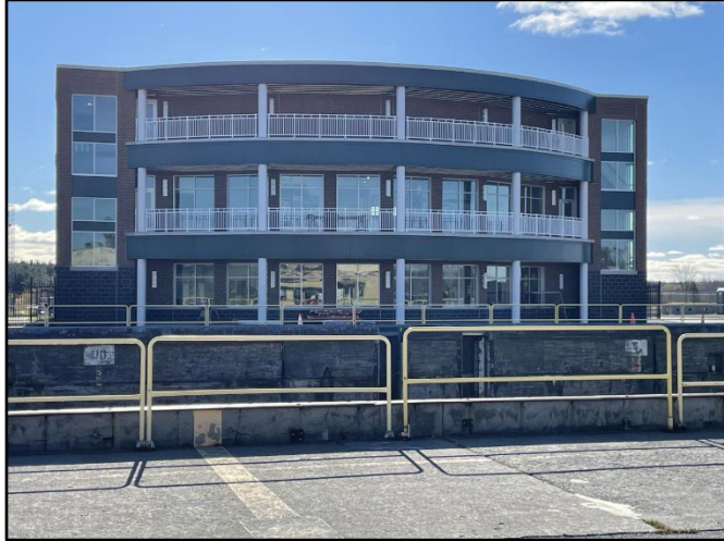
New Seaway Visitor Center at Eisenhower Lock in Massena, New York
