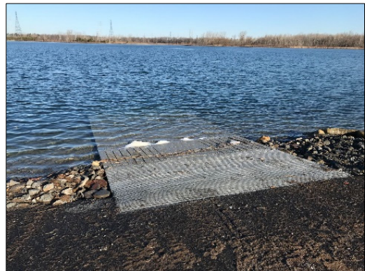
The new GLS Marine Base boat launch ramp.
