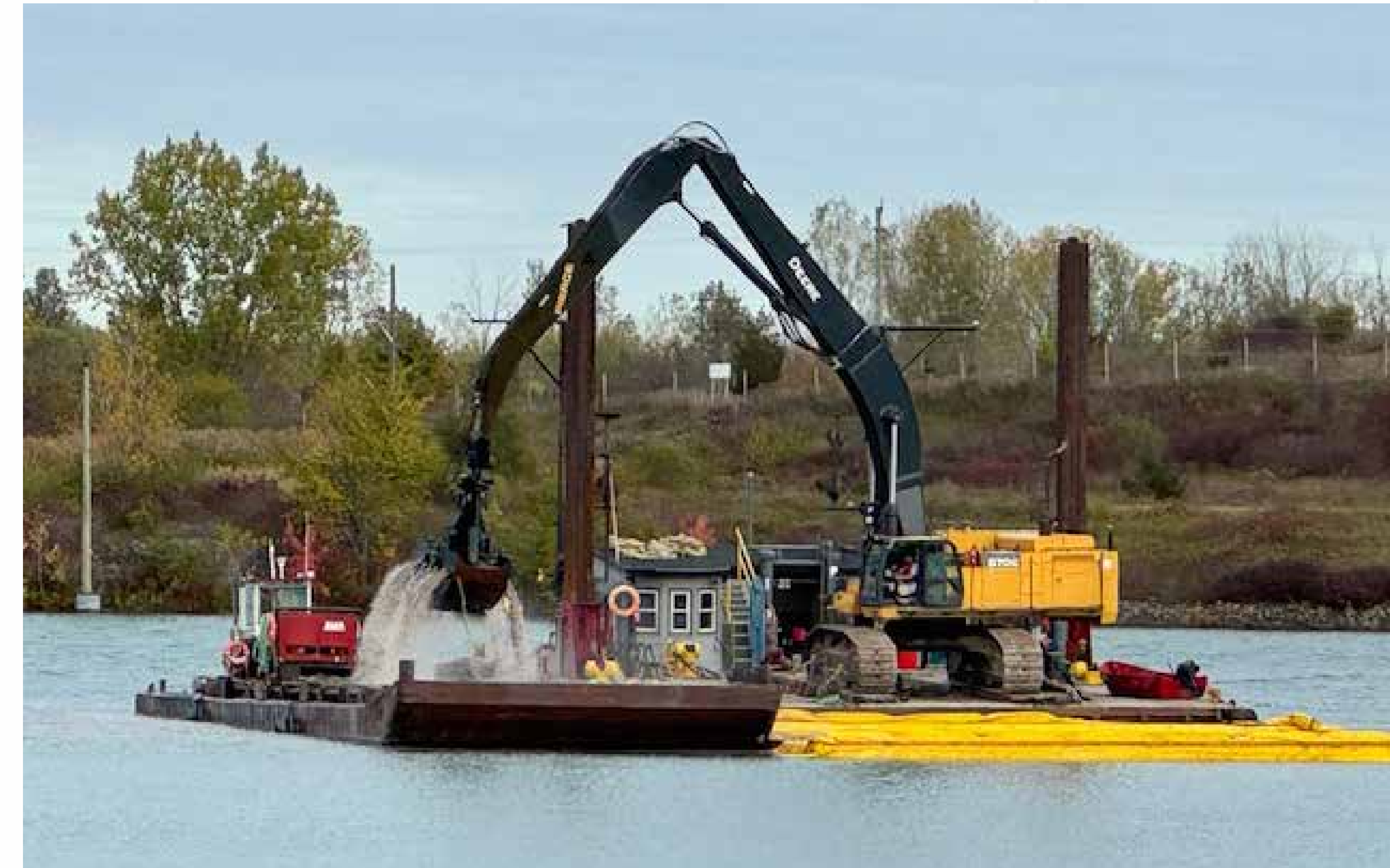
Dredging at Wharf 10, Welland Canal
