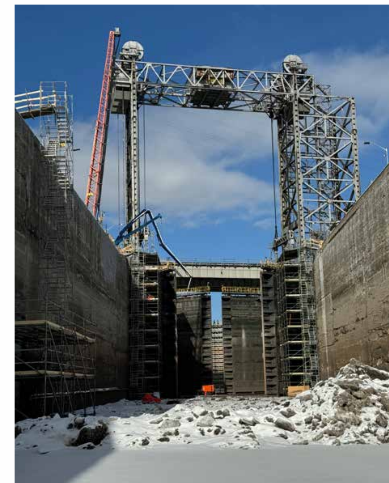
Rehabilitation work at St. Lambert Lock
